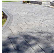
PERMEABLE PAVER DRIVEWAY
